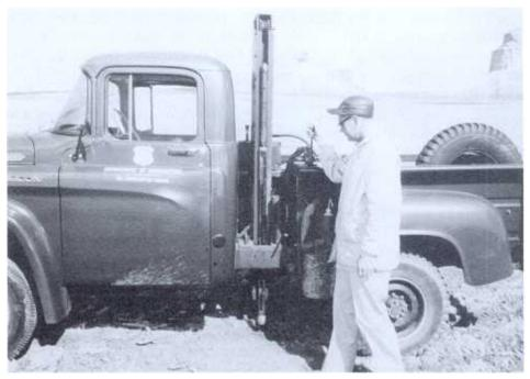
Truck with probe to withdraw cylindrical cores of soil about 5 cm in diameter and 1.5 m long. The probe is forced into the soil and withdrawn by a hydraulic pump powered by the truck motor. Power probes are of various lengths with most between 1 and 2 m. USDA photograph.
