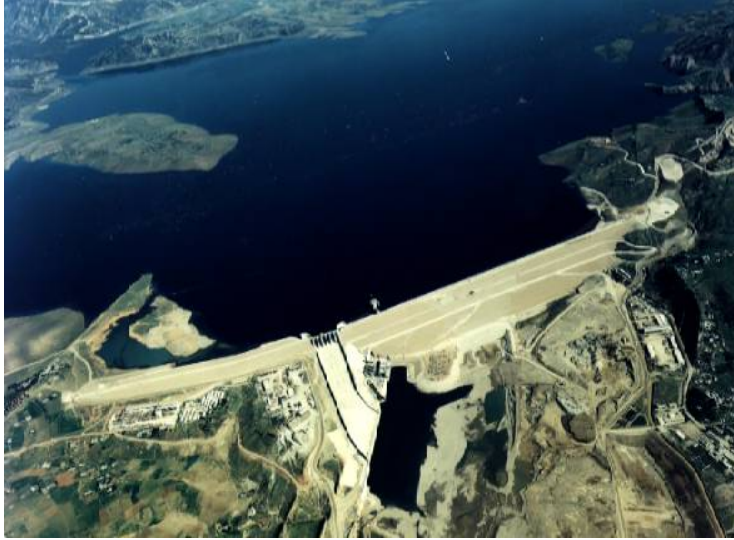
Figure 31 Al Wahda dam, Sebou basin
