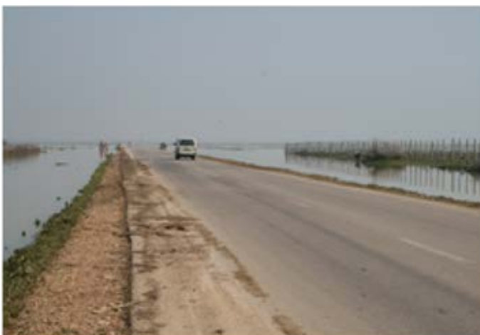
Figure 17 Flooding in the Sebou basin during 2009-2010 (ABHS 2010)
